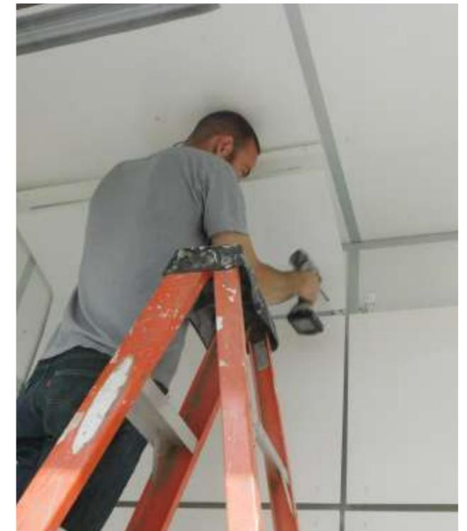
Install (Left Top Baffle A) to (Back Wall A) and (Ceiling Panel A).
