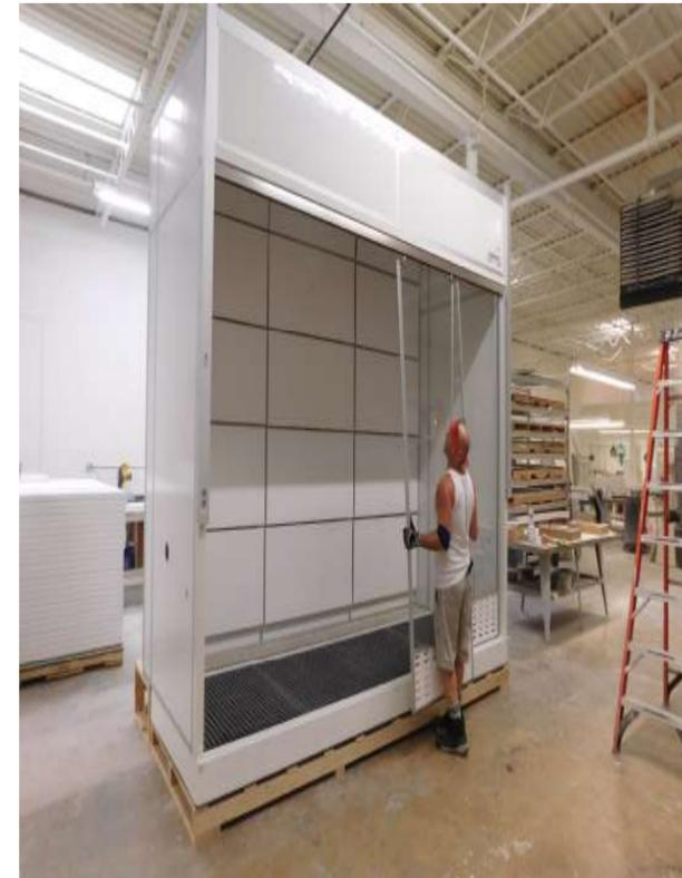
Install the (Sliding Door L) into the Door Frame .
