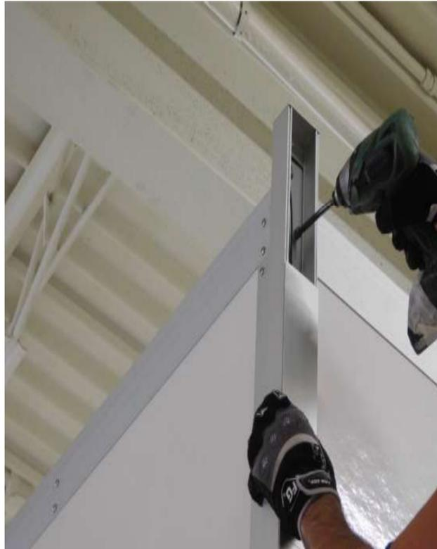
Install Left and Right (Electrical Chases), to front corners of hood. Secure with provided #10 sheet metal screws.
