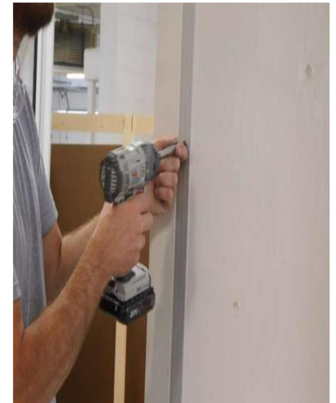
Secure from right and left sides with provided #10 sheet metal screws, and Bolts.
