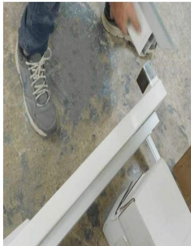
Assemble (Steel Door Frame) by sliding header into
