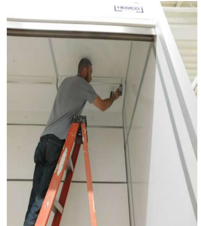
Install (Right Top Baffle C) to (Back Wall C) and (Ceiling Panel C).
