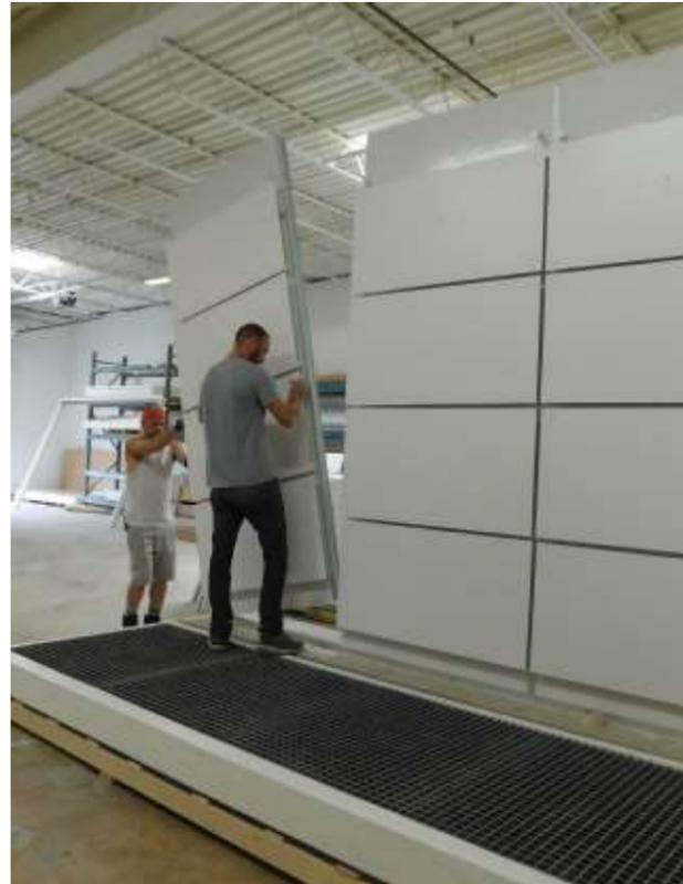
Attach Panel (Left Back Wall A) to (Center Back Wall B).
