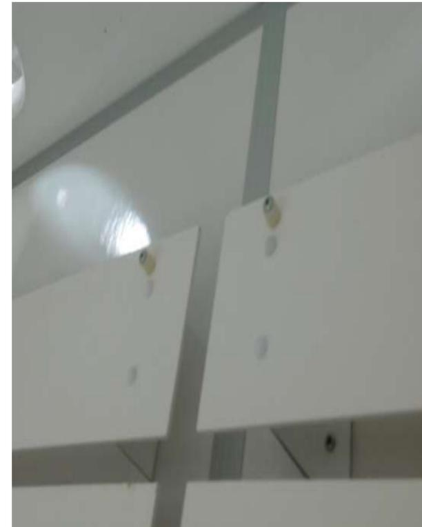
View of top of Rear Baffles. Remove spacers and screws, and use to install upper Baffles.
