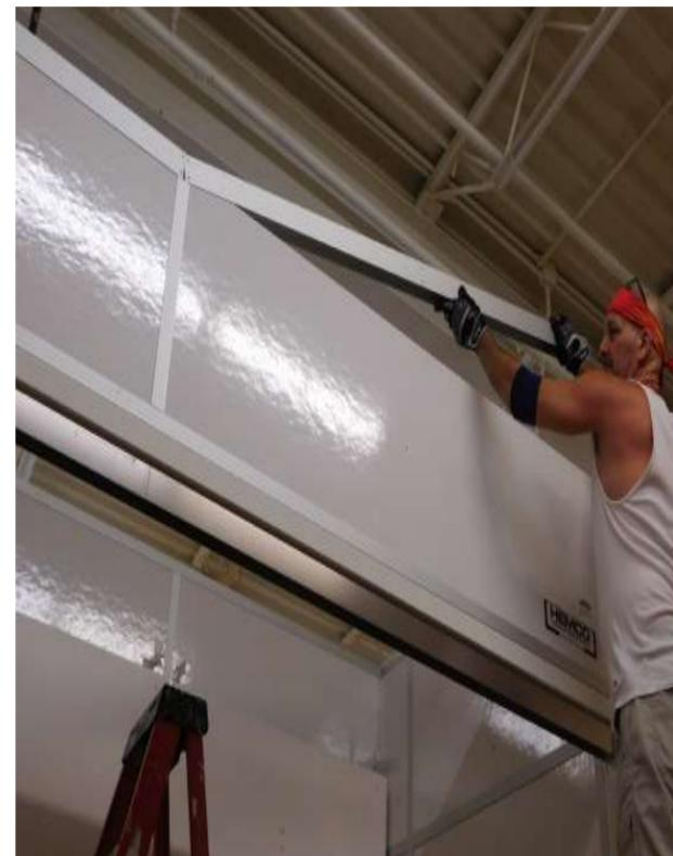
Install (2) Aluminum channels to top of Front wall.
