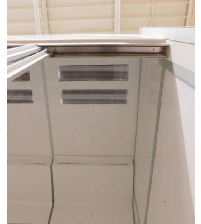
Note: Holes for Duct work are located toward the back of the Hood, and Lighting is located toward the front of the hood.
