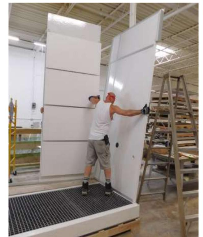
Attach Panel (Right Side Walls D / E) to (Right Side Back Wall C). Secure From back with #10 sheet metal screws.
