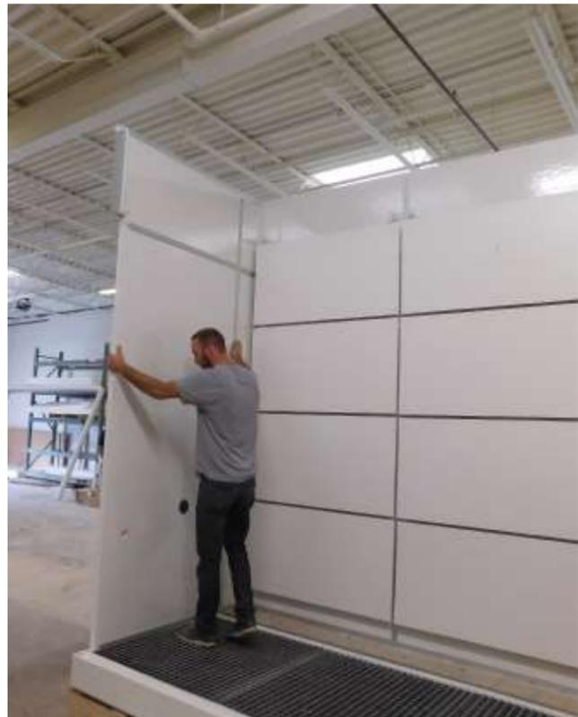
Attach Panel (Left Wall H / F) to (Left Back Wall A).
