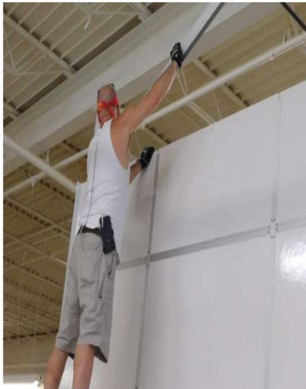
Attach Aluminum Channels (2) to top of Back wall.
