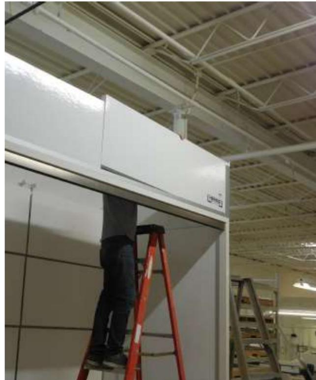
Attach (Right Header I) into track above (Steel door frame I) insert aluminum channel between headers.
