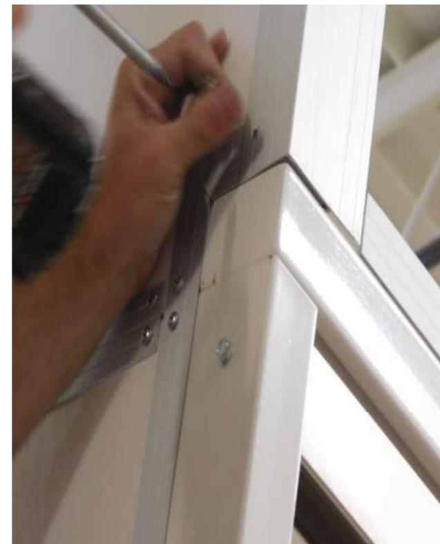
Install aluminum angle to left and right walls above door frame. Secure with provided #10 sheet metal screws.
