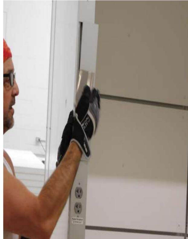
Snap cover onto front of Electrical chases.
