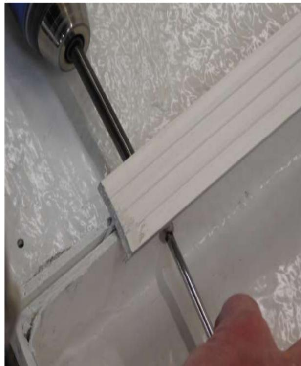
Install: Machine screws and locknuts to hold the ceiling panels together.
