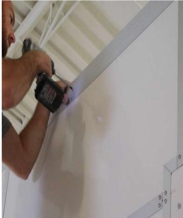
Secure Aluminum Channels to Ceiling Panels on all four sides with provided #10 sheet metal screws.
