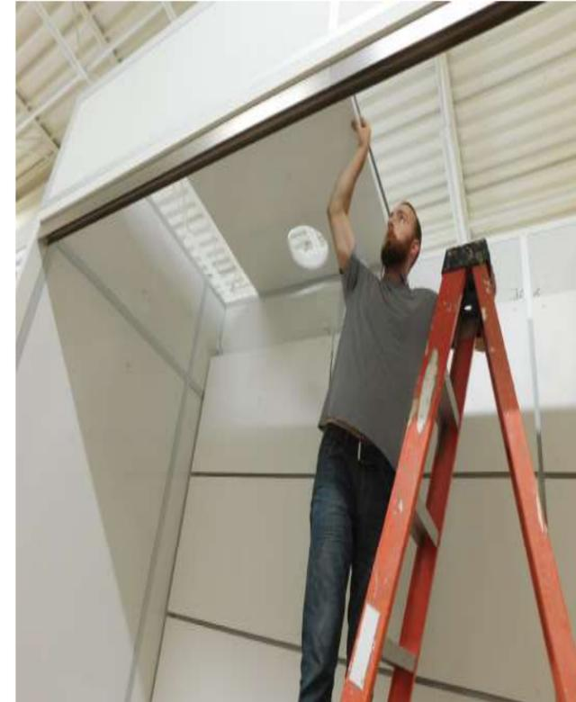
Install (Left Ceiling Panel A) into Aluminum channels. Install Aluminum channel between Ceiling Panels.
