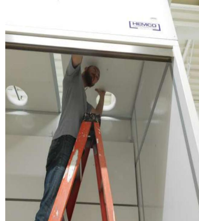
Install (Right Ceiling Panel C) into Aluminum channels.
